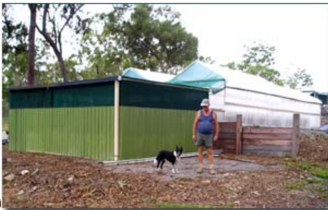
"The Large System" The fish shed in the foreground and the greenhouses above and behind.
