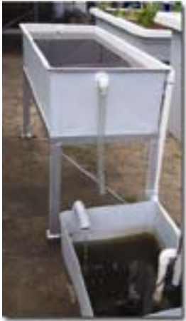
ABOVE: The overflow and return pipe to the sump can be seen.
